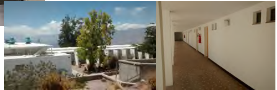
Dormitory repainted inside & out, roof repaired
