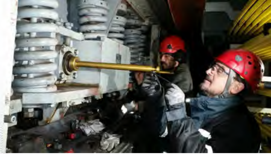
Precise alignment of dome trucks to increase bearing life
