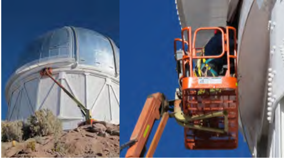
Replacing failed bearings on dome trucks
