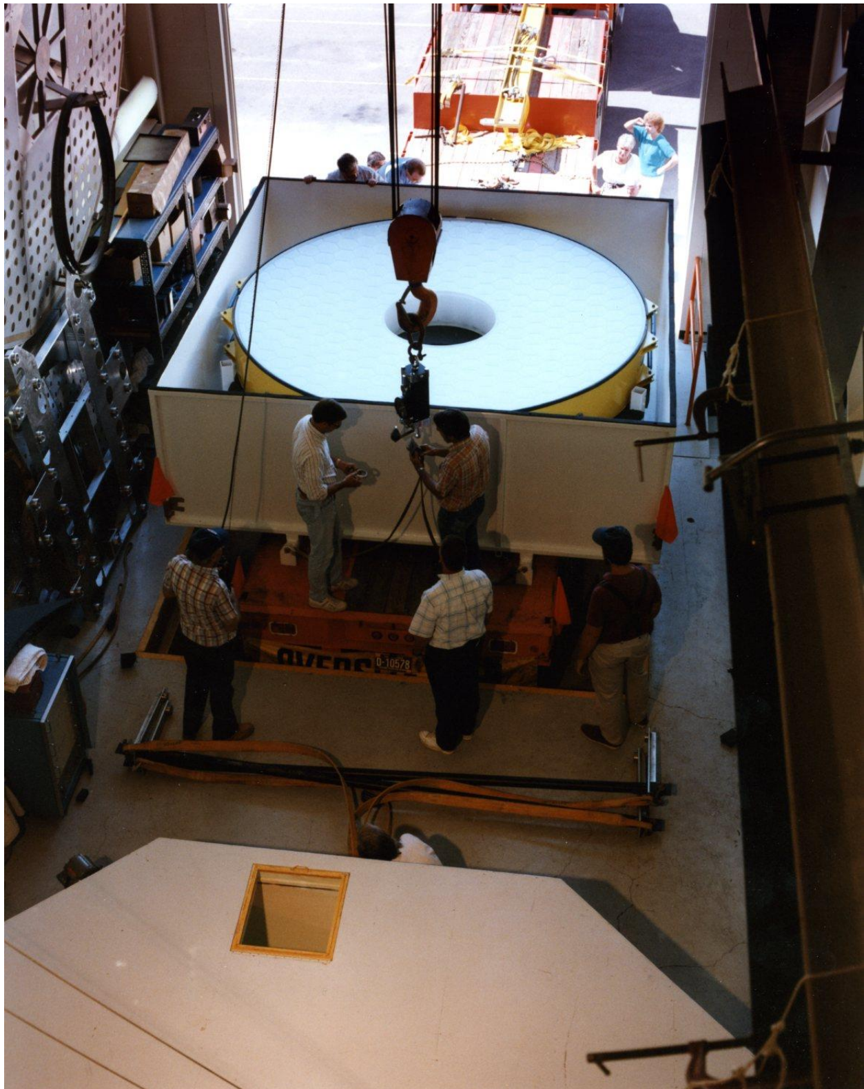
Caption: Larry Stepp and Dave Dryden detaching cables from the hydraset suspended from the crane
