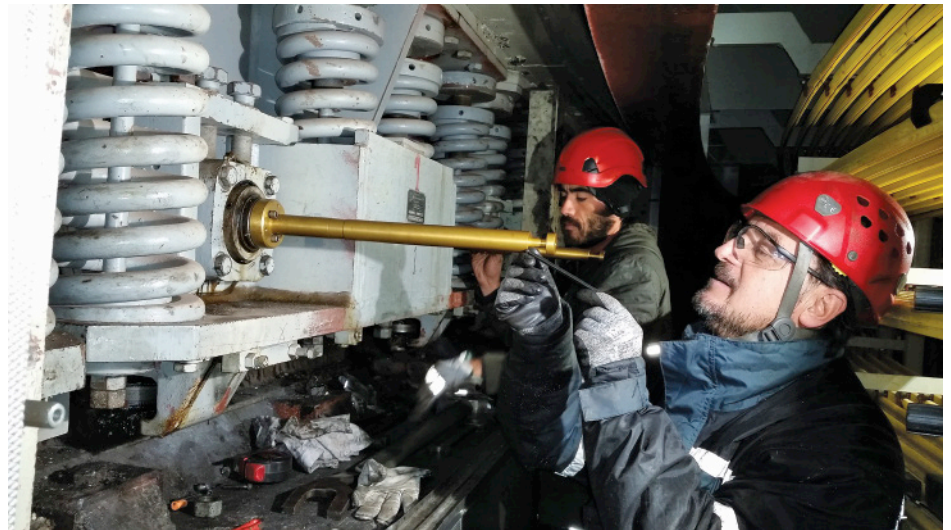
Figure 2: Telescope mechanics Jorge Briones and Christian Diaz work to measure the alignment of one of the trucks for the Blanco telescope dome. Proper operation requires quite precise adjustment of the 2,100 kg truck. (Image credit: Andrés Montané, NOAO/AURA/NSF.)
