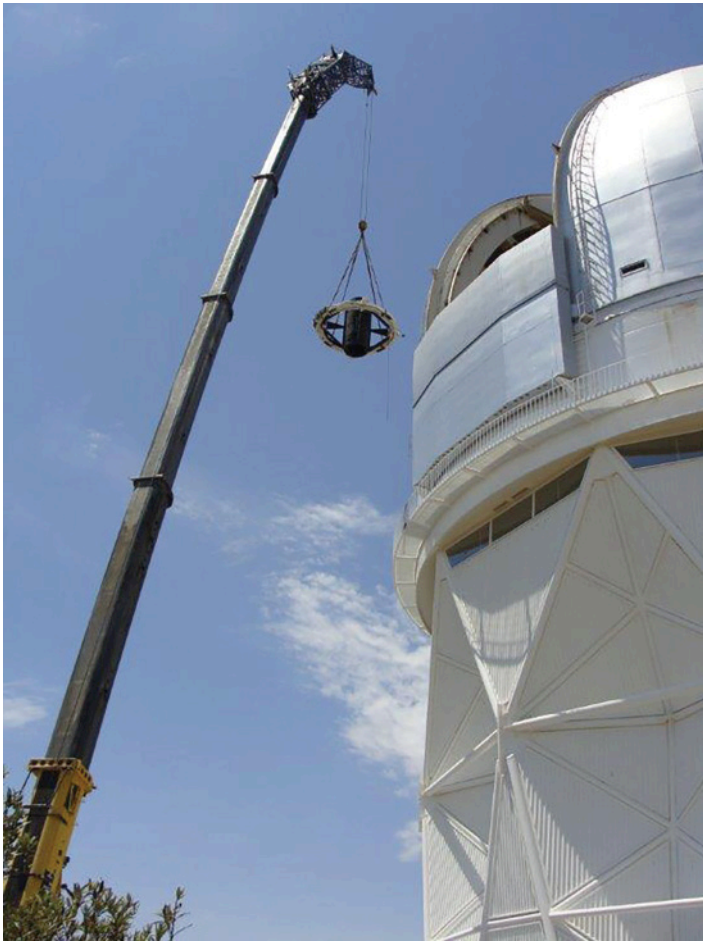
Figure 1. The old top ring and prime focus cage being lifted out of the Mayall telescope in June 2018, to be replaced by the DESI top ring and corrector. (Credit: D. Sprayberry/NOAO/AURA/NSF)
