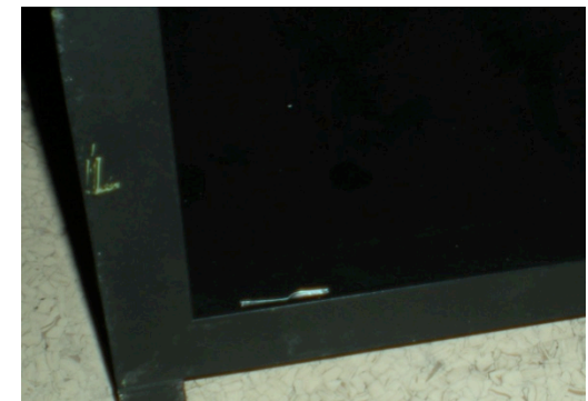
Steel cover mounted around grating onto seal
