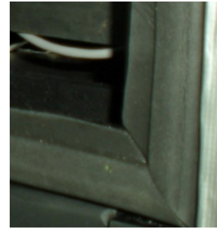
Close-up view of seal
