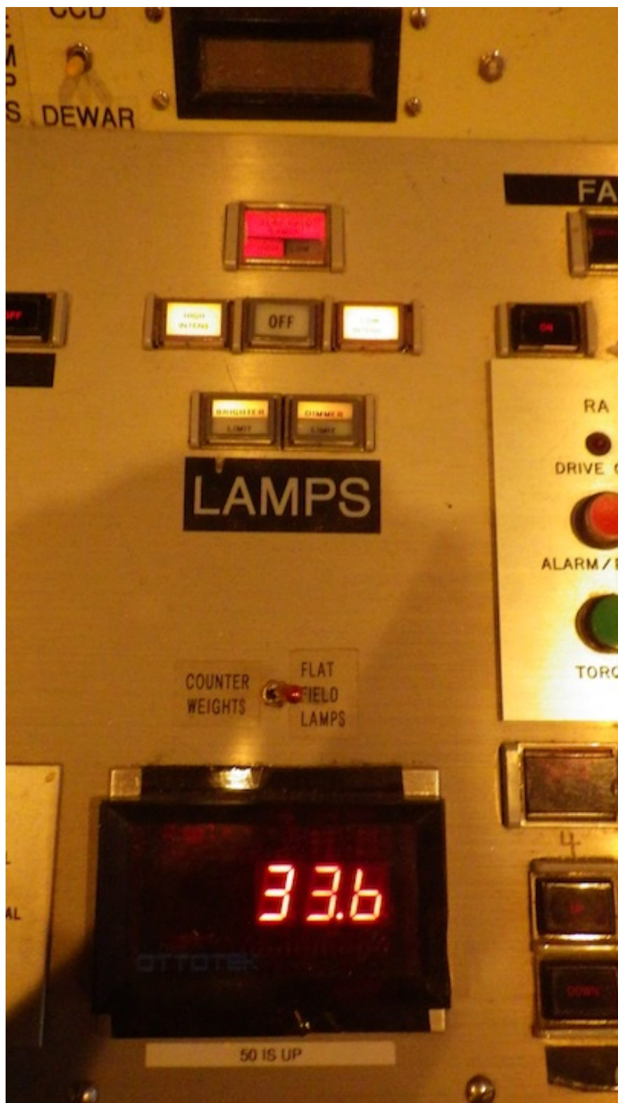
Fig. 34. Dome flat lamp control buttons, toggle switch, and brightness display.
