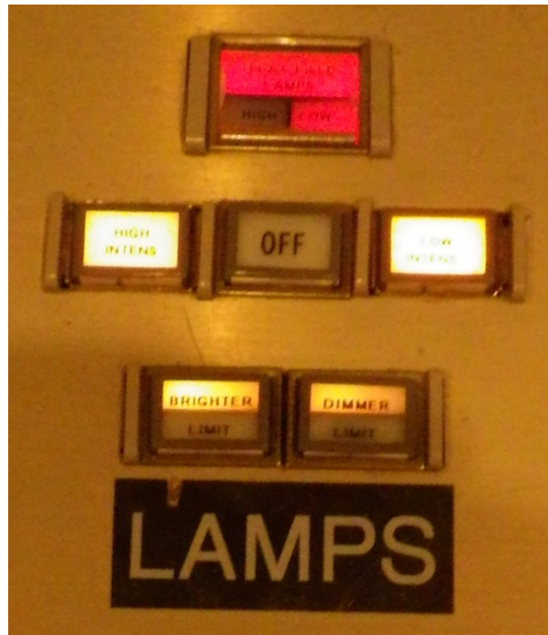
Fig. 37. Dome flat lamp pushbuttons with low lamps selected.
