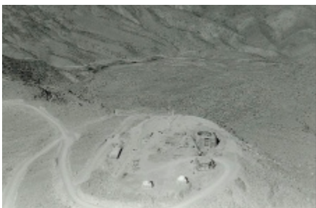
Figure 2: The Cerro Tololo construction site in 1963.
