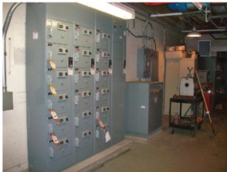
Figure 15: Old (left) and new (right) electrical distribution control panel in the main Tucson building. (Image credit: Kate Foster, NOAO/AURA/NSF.)
