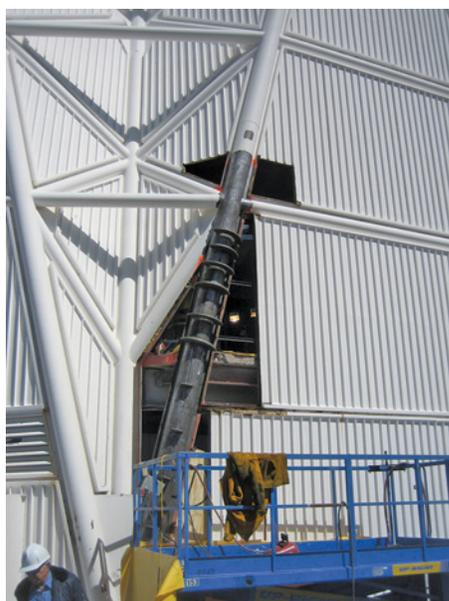
Figure 3: Repair of Mayall 4-m telescope column with strongbacks. (Image Credit: Kitt Peak Facilities, NOAO/AURA/NSF.)
