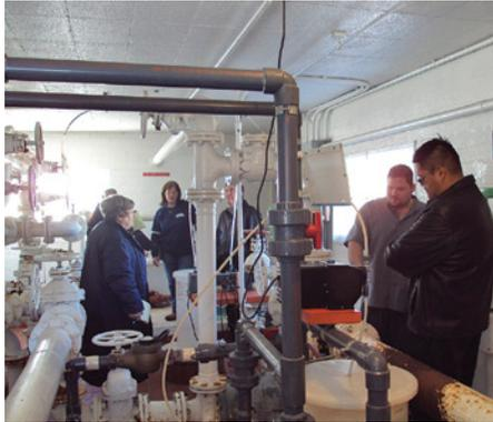
Figure 11: Kitt Peak pump house for the water distribution system. This facility will undergo a major renovation in FY12. The project has been developed and is out for bid to external contractors (some of whom are shown here reviewing the existing pumps, piping, and filters that will be replaced). The total project is valued at approximately \$1M. (Image credit: Kate Foster, NOAO/AURA/NSF.)
