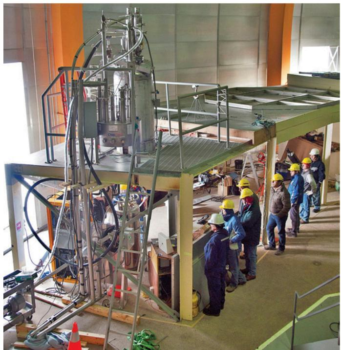
Figure 3: Liquid Nitrogen system for cooling DECam. The system is installed in and on top of the old console room in the Blanco dome. (Image credit: Tim Abbott, NOAO/AURA/NSF.)
