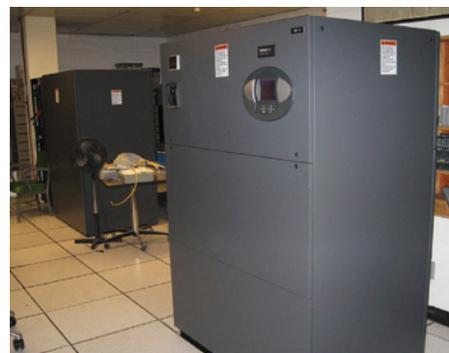
Figure 13; New Tucson main computer room air handling unit. (Image credit: John Dunlop, NOAO/AURA/NSF.)
