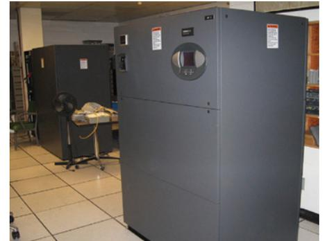
Figure 13; New Tucson main computer room air handling unit. (Image credit: John Dunlop, NOAO/AURA/NSF.)
