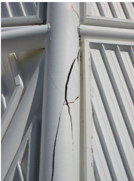
Figure 1: Cracked column on Mayall 4-m telescope. (Image credit: Kitt Peak Facilities, NOAO/AURA/NSF.)
