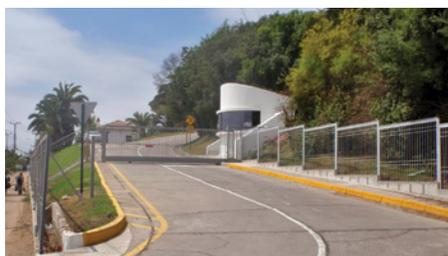
Figure 10: Before (left) and after (right) views of the main entrance to the La Serena base facility, which includes CTIO, SOAR, Gemini, and soon LSST buildings. The new main gate was needed because the city installed a traffic light just below, but without a signal for the observatory entrance! The recessed gate allows traffic to enter without stopping on busy Calle Cisternas. (Image credit: Enrique Figueroa, NOAO/AURA/NSF.)
