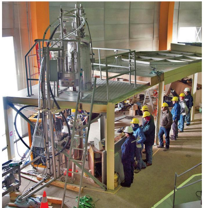
Figure 3: Liquid Nitrogen system for cooling DECam. The system is installed in and on top of the old console room in the Blanco dome. (Image credit: Tim Abbott, NOAO/AURA/NSF.)
