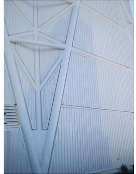
Figure 4: Finished repairs of cracked column on Mayall 4-m telescope. (Image Credit: Kitt Peak Facilities, NOAO/AURA/NSF.)
