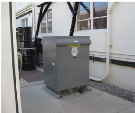
Figure 14: Old transformer at the Tucson main facility being removed (left). Installed new transformer (right), which is part of the electrical distribution system upgrade. (Image credit: Kate Foster, NOAO/AURA/NSF.)
