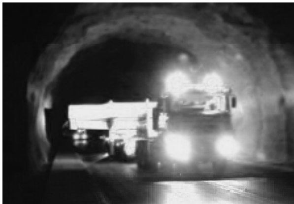
Passing through the Puclaro Dam Tunnel.
