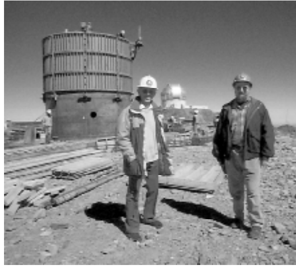
Malcolm Smith and Steve Heathcote stand in front of the pier that will support the SOAR telescope. In mid-April 2000 the concrete work for the lower half is complete, with the forms in place to the full height of the pier. The Gemini South dome is seen in the background.
