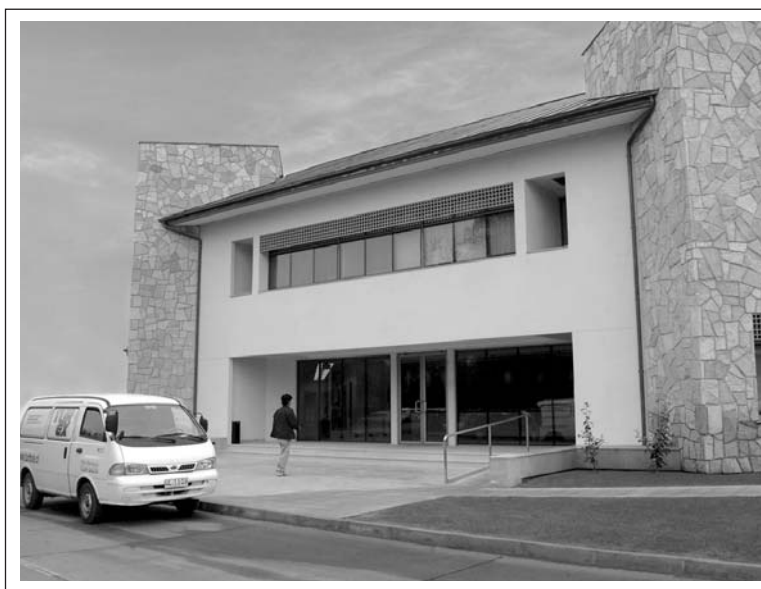
The front entrance of the Gemini South Base Facility showing the locally quarried stone facade and Chilean copper roof. See additional images of this new facility on the opposite page.
