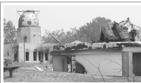
Rear view of the administration building and remnants of the 50 inch telescope on Mt. Stromlo after the January fire. Photo courtesy of Matthew Colless, RSAA, ANU.
