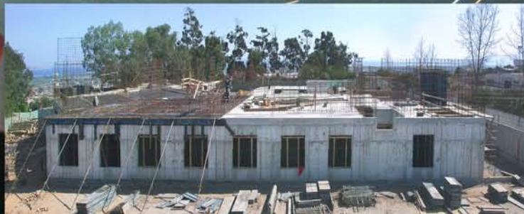
Gemini South Base Facility construction late April, 2002. Photo by: Antonieta Garcia
